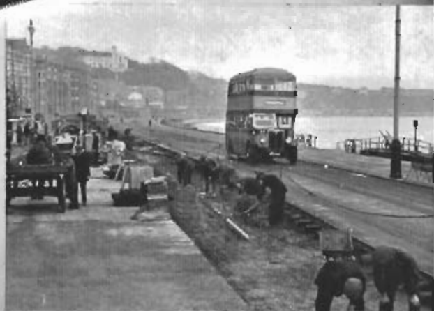
Re-surfacing the central promenade, Douglas L.O.M. to provide a practically skid-proof face for next year's Mannin Races.
