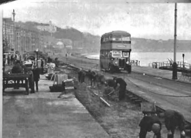
Re-surfacing the central promenade, Douglas L.O.M. to provide a practically skid-proof face for next year's Mannin Races.
