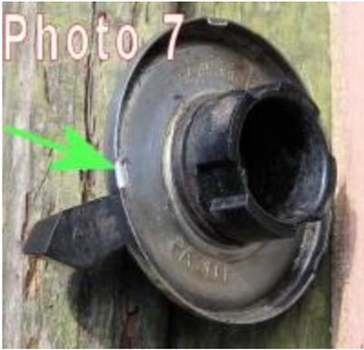
**Photo 7** - these three lugs are placed asymmetrically around the rim, they can only be fitted correctly to the moulded base one way, there are three openings in the moulded base rim (**photo 8 - arrowed B**) for these face plate lugs to be pushed down through, the face plate has to be turned anti-clockwise for about ½” were the lugs should find a ‘safe’ dip (**photo 8 - arrowed A**) to stop the face plate turning.
